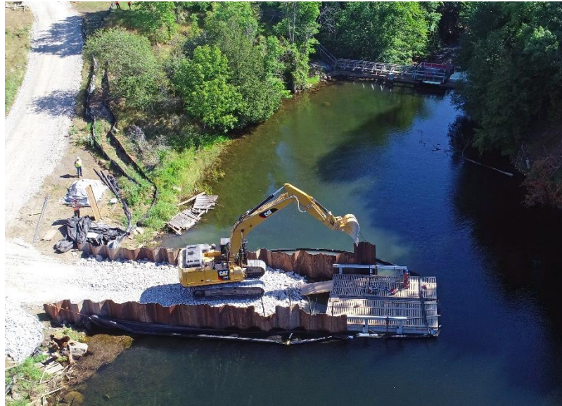
Contractor setting up the cofferdam
